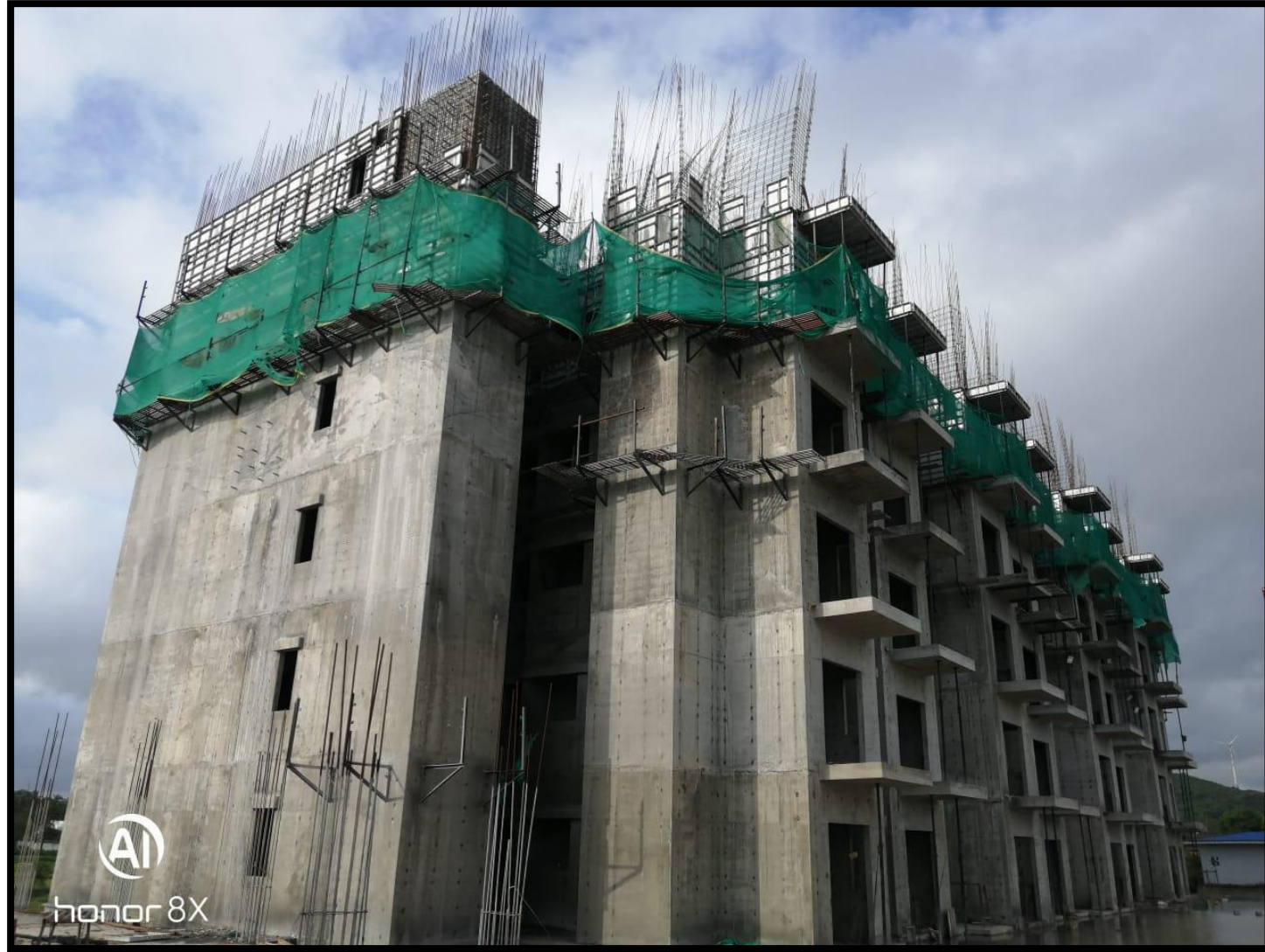
5th FLOOR ALUFORM WORK IN PROGRESS
