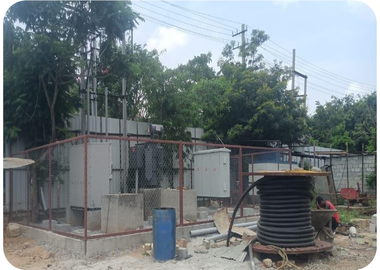
Transformer yard installation work in progress
