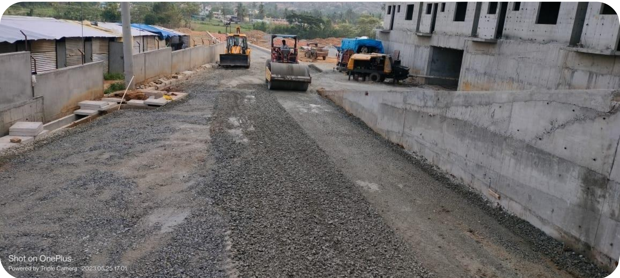
Tower C East side drive way base preparation work in progress
